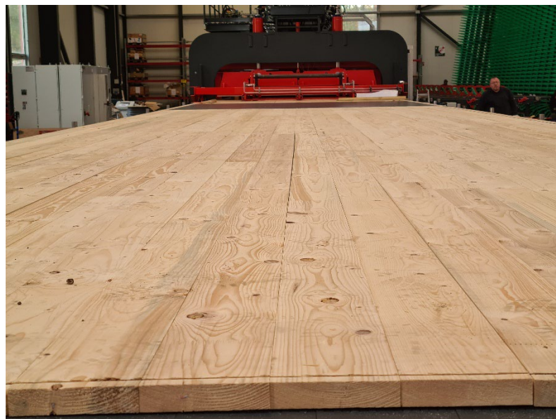
Length layer with layer stabilization system in preparation for the pressing process
